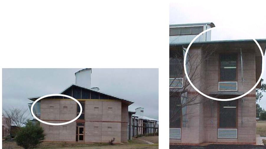
Figure 2 Westerly and northerly views respectively of the office studied
