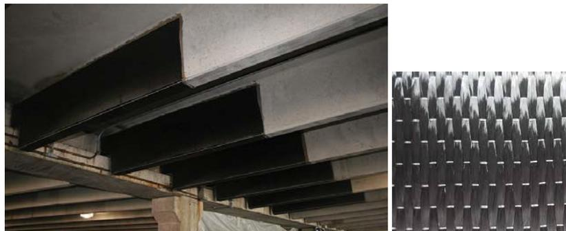
Figure 1 Structural strengthening using CFRP
