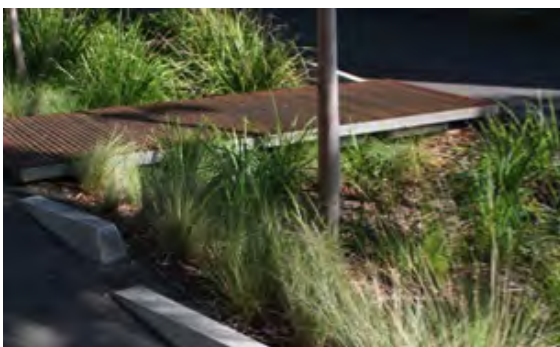
Figure 6.18: Showing scenario 1: at grade (WSUD) road median, Victoria Park Sydney.
