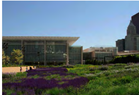
Figure 5.18: Lurie Garden's sophisticated and low maintenance perennial planting (on slab).
