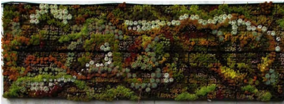
Figure 6.20: Succulents have very low water, nutrient and maintenance needs, but require high light levels, and are more vulnerable to wind and hail damage (not issues if indoors in sealed environment).
