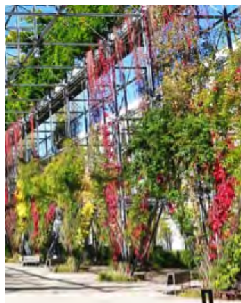
Figure 6.22: Showing scenario 3: climbing plants on stainless wire support system. MFO Park, Switzerland.
