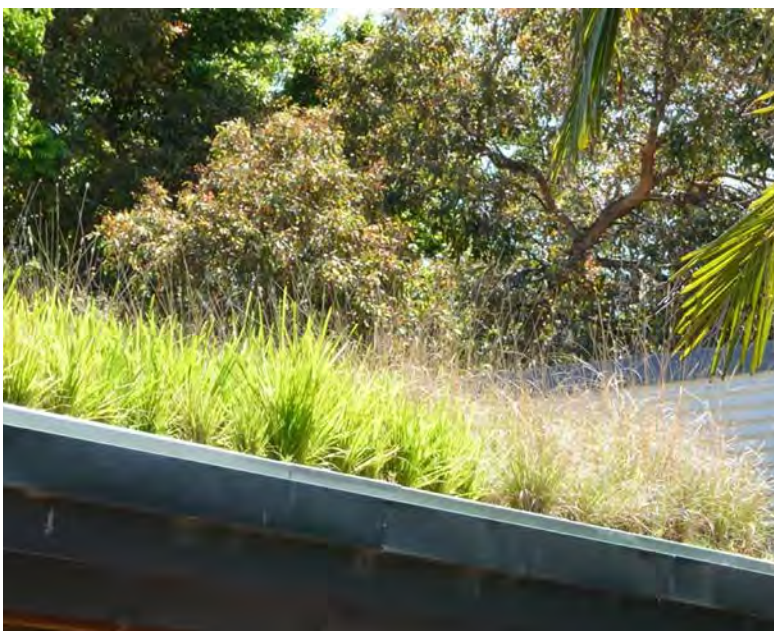
Figure 7.1: Key biophilic design elements, green roofs cool the air, provide retention for stormwater run-off, add to biodiversity – and offer potential as living laboratories for researching climate change response. Source: Downton
