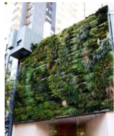
Figure 6.23: Showing scenario 4: vertical green wall system at Triptych Apartments, Southbank Melbourne.
