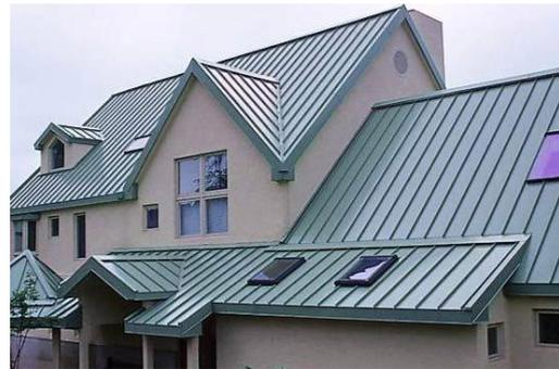
Fig. 1 Long Run Metal Roof
