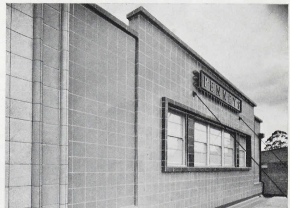
SHOWING TREATMENT AROUND WINDOWS AND GLAZED TERRA-COTTA COPING TO PREMISES AT RYDE, N.S.W.
