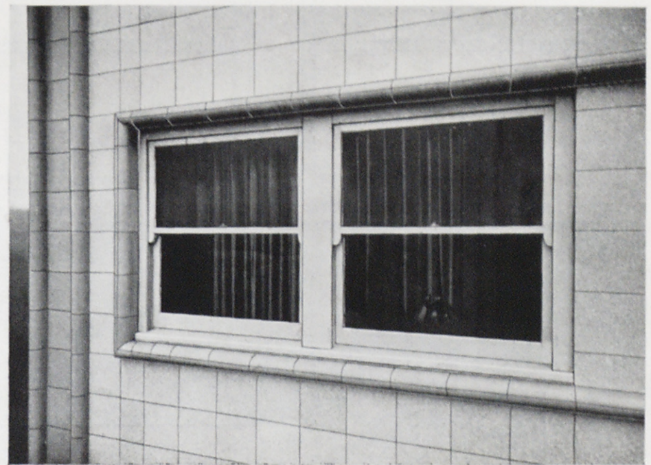
VERTICAL FEATURE AT SIDE AND AROUND WINDOWS ARE CUT FROM THE STANDARD BLOCK ILLUSTRATED ON NEXT PAGE.
