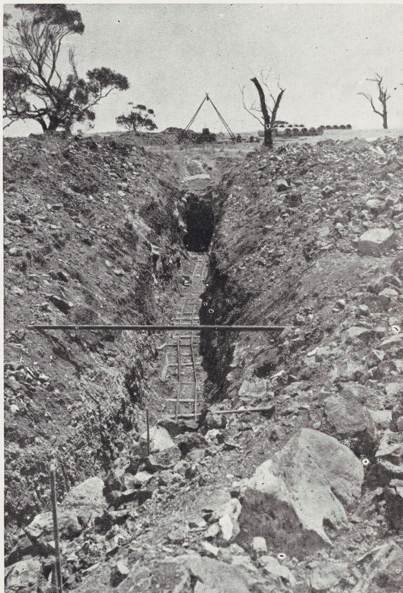
CHANNEL EXCAVATION AND PIPES AT TUNNEL APPROACH
