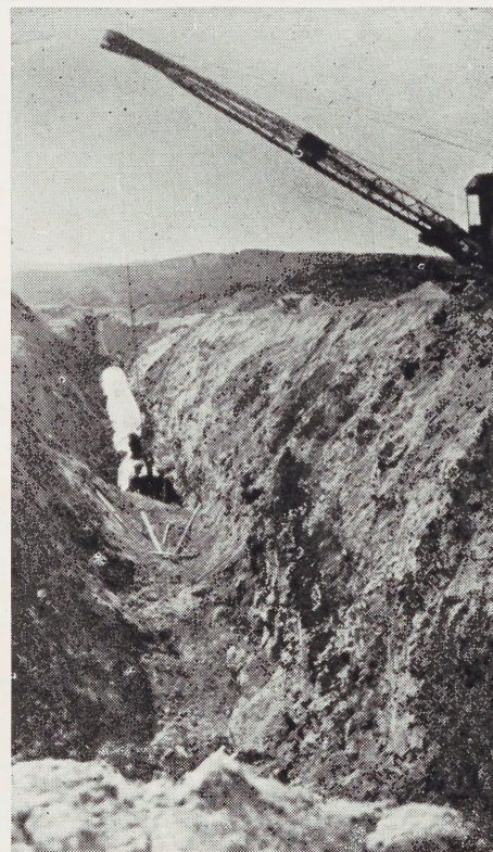
CHANNEL EXCAVATION AND PIPES AT TUNNEL APPROACH
