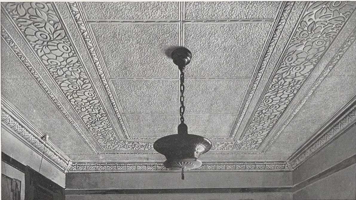
The complete Wunderlich Metal Ceiling—Suite Nos. 1623-1624—installed and decorated.
