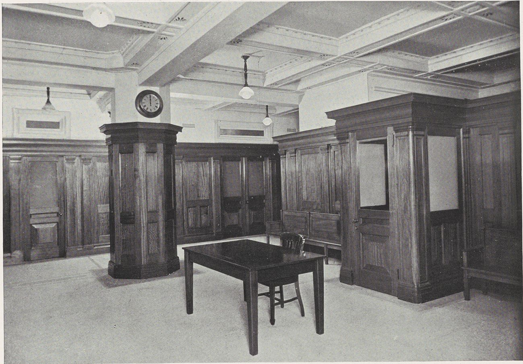
Wunderlich Steel Cornice and Girder Casing, Government Savings Bank of New South Wales, Sydney.
