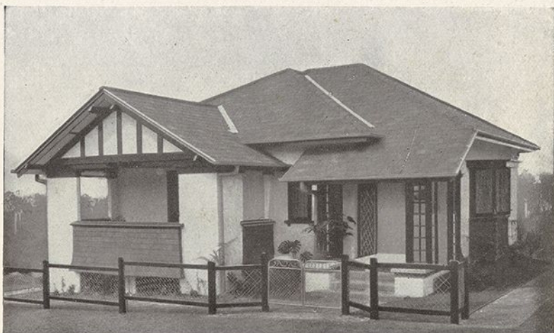
"Fibrolite" Asbestos Cement Dwelling with Exterior Walls roughcast. Ground Plan for this cottage supplied on request.
