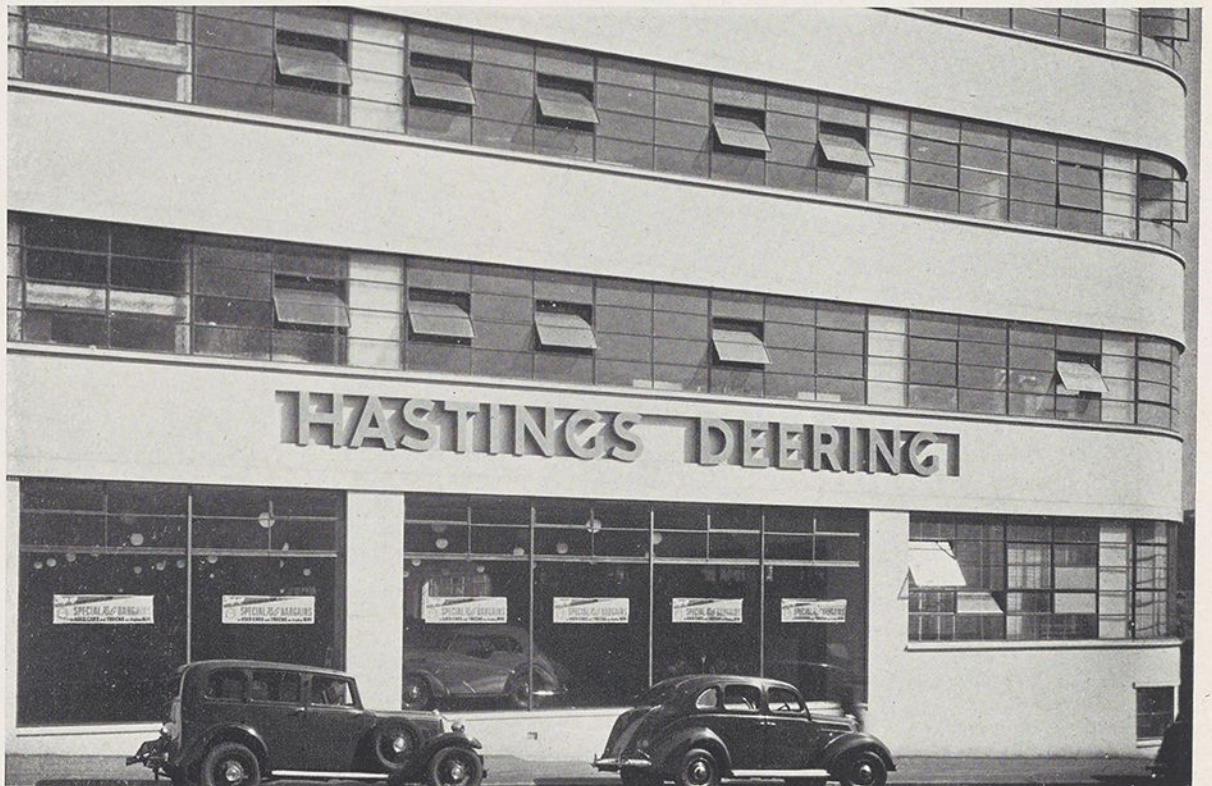
BUILT ZINC LETTERS, 33" HIGH. FACES AND SIDES PAINTED BUFF AND SANDED TO REPRESENT STONE ARCHITECT: SAMUEL LIPSON BUILDERS: HOWIE MOFFAT AND CO. PTY. LTD.
