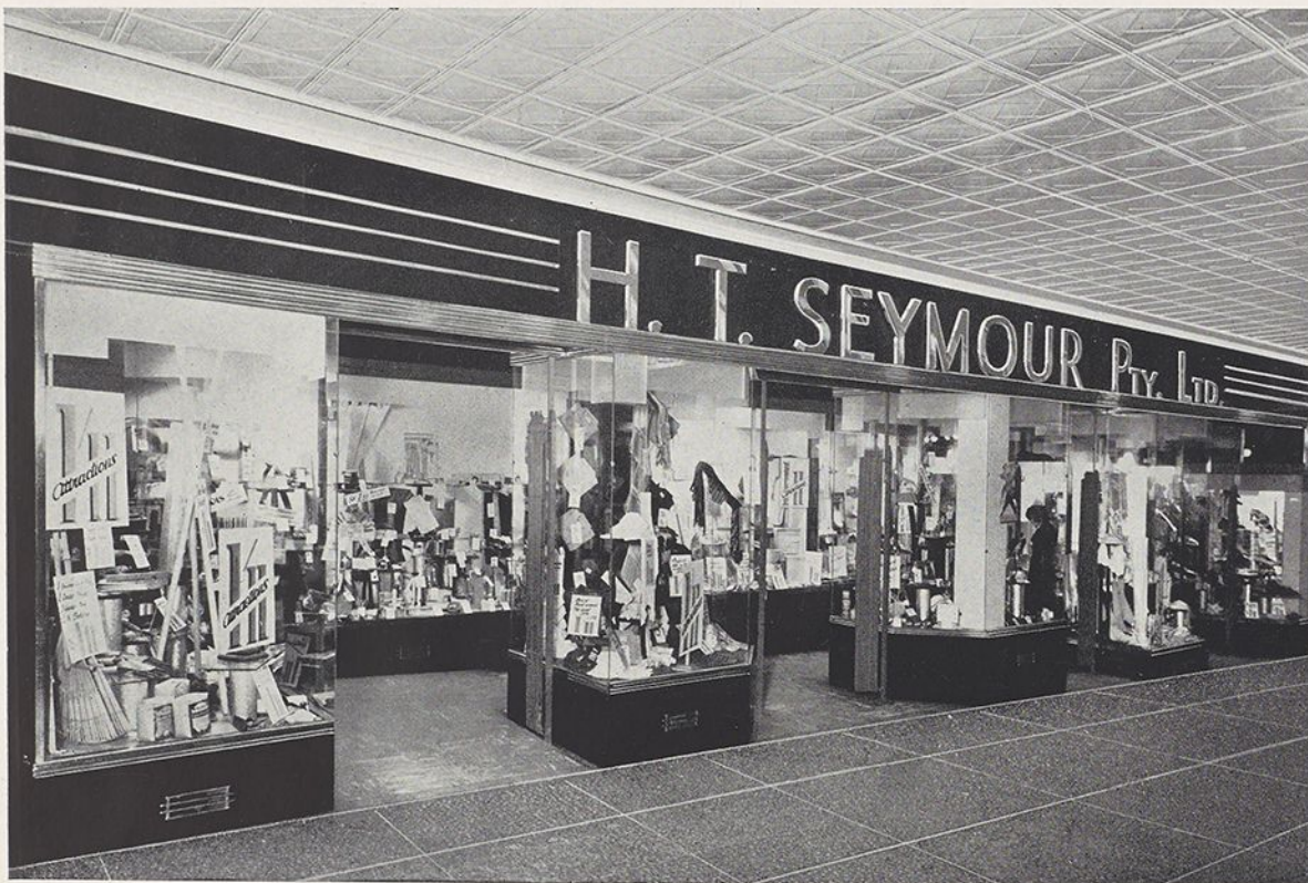
BUILT MONEL LETTERS, 18" AND 9" HIGH. FACES AND SIDES POLISHED FINISH ARCHITECT: H. W. BLACKET CONTRACTORS: ARMSTRONG BROS. PTY. LTD.
