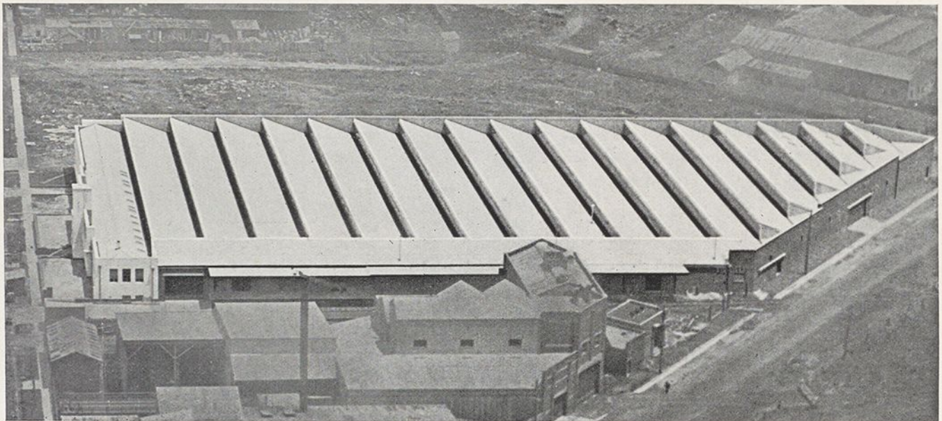
DEEP CORRUGATED DURABESTOS ROOFING to the Southern Can Company's new building, West Footscray, Victoria. Area: 85,000 sq. ft. Architects: Oakley & Parkes. Contractors: Hansen & Yuncken.
