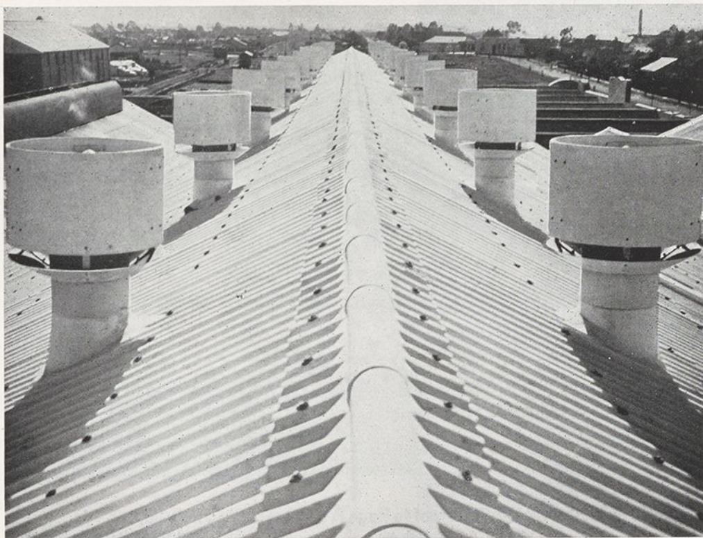
Another view of the roof to the Australian Paper Mills showing some of the thirty-six 16" diam. Durabestos Roof Ventilators. One hundred and six Durabestos Skylights were also used on this roof.
