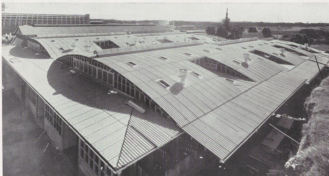
WUNDERLICH DEEP CORRUGATED DURABESTOS ROOFING to the Pig Pavilion, Royal Agricultural Society's Show-ground, Sydney. The Durabestos Sheets, Skylights and Roof Slope Bases are curved to the contour of the Patent (S.S.) Roof Truss.
