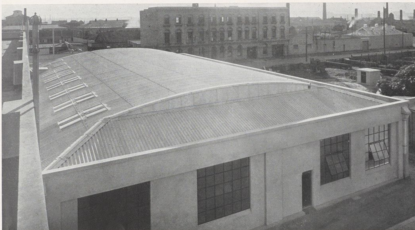
WUNDERLICH CURVED DEEP CORRUGATED DURABESTOS ROOFING to Messrs. BATES (AUST.) LIMITED FACTORY AT ROSEBERY, N.S.W. The Durabestos Sheets are curved to the contour of the Patent (S.S.) Roof Truss. Area: 7,800 sq. ft.
