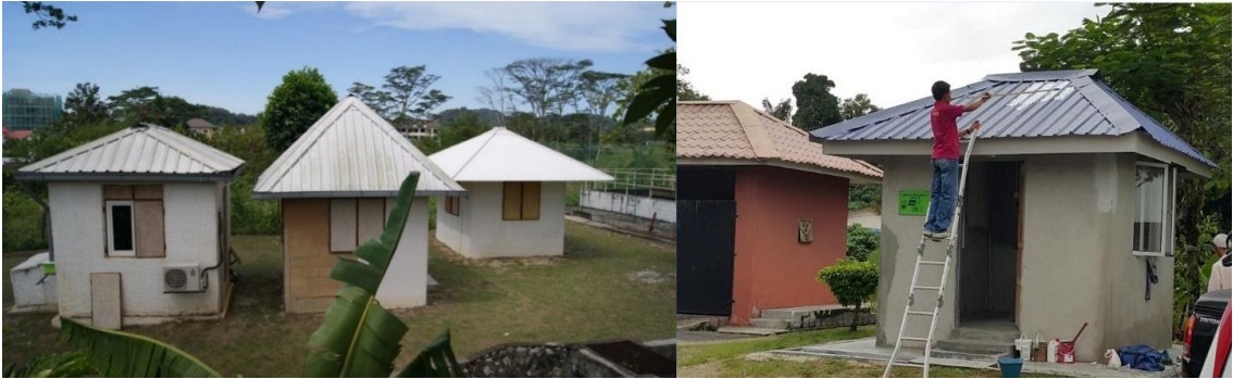
Figure 4: 3 Green & Energy Efficient Passive Buildings based on the Passive House design (left) and the (later improved coated) conventional house (right) at the Triple Green Mock-Up Building Park with the same positioning on UniKL’s premises at Gombak/ Kuala Lumpur
